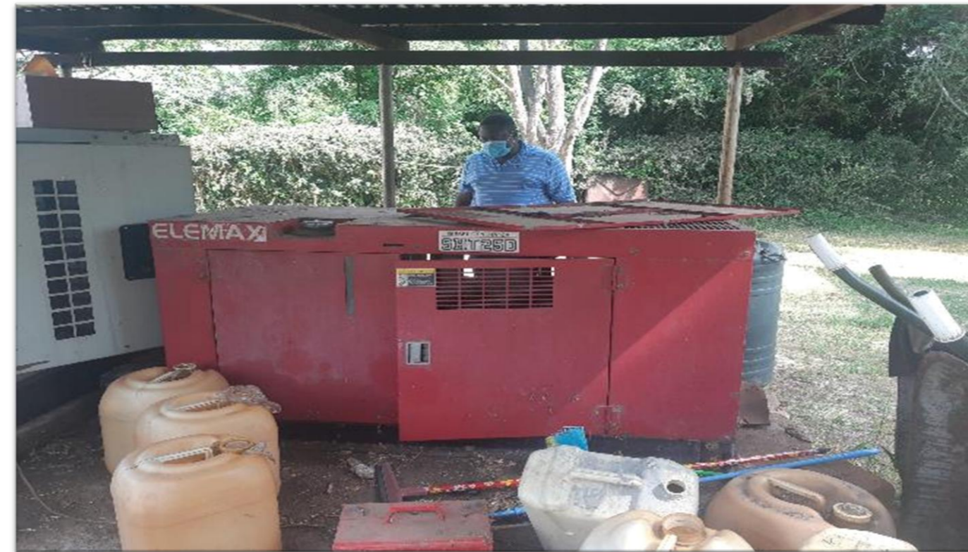
PDP/GIZ/IRC-Moroto: Site assessment and load profile measurements at 10 sites.
