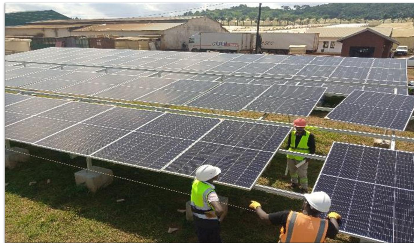
200 kWp Solar PV solution, 200 kWh solar back-up at Jambo Roses ,Nakawuka.
