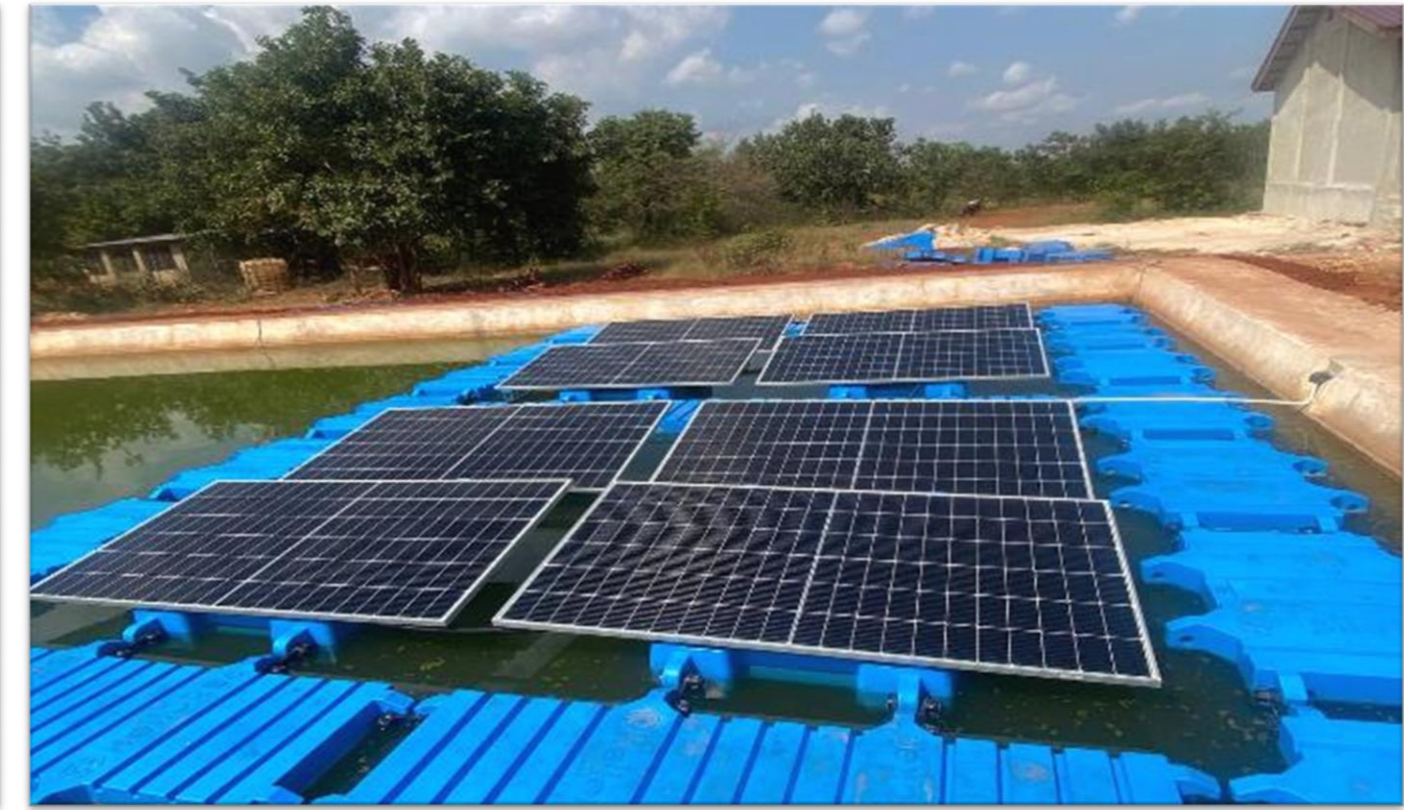
22 kWp and 57 kWh solar system with back up at Sustainable Agriculture Tanzania in Morogoro.
