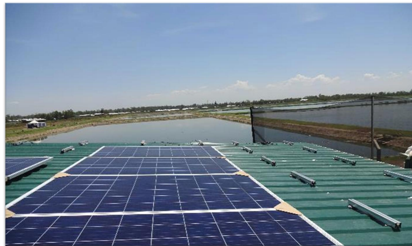
20 kWp and 19kWh solar system with back up at Department of Agriculture Kisumu Kenya.
