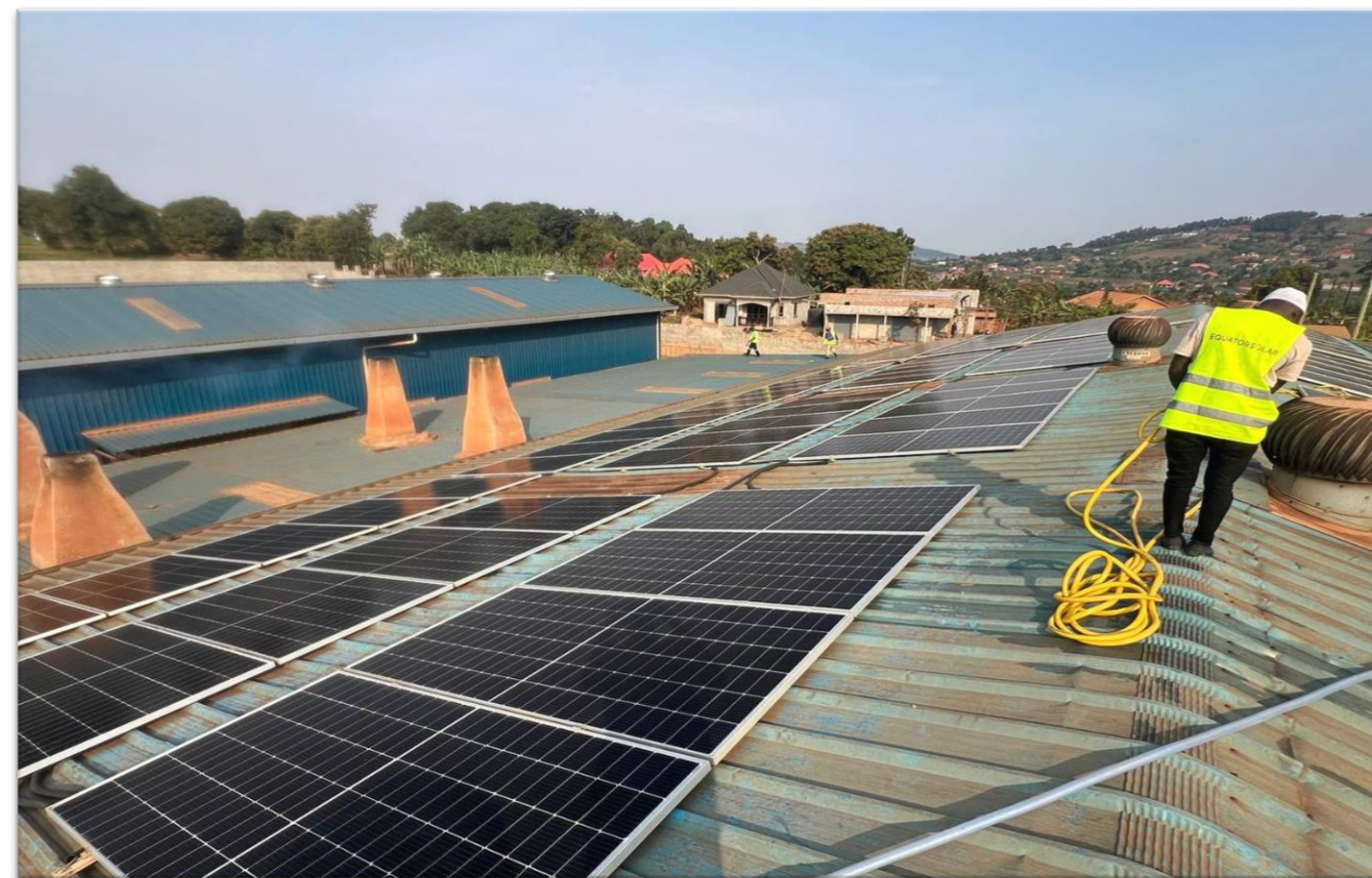
Kyamuhunga Tea Factory: Solar panel cleaning taking place.
