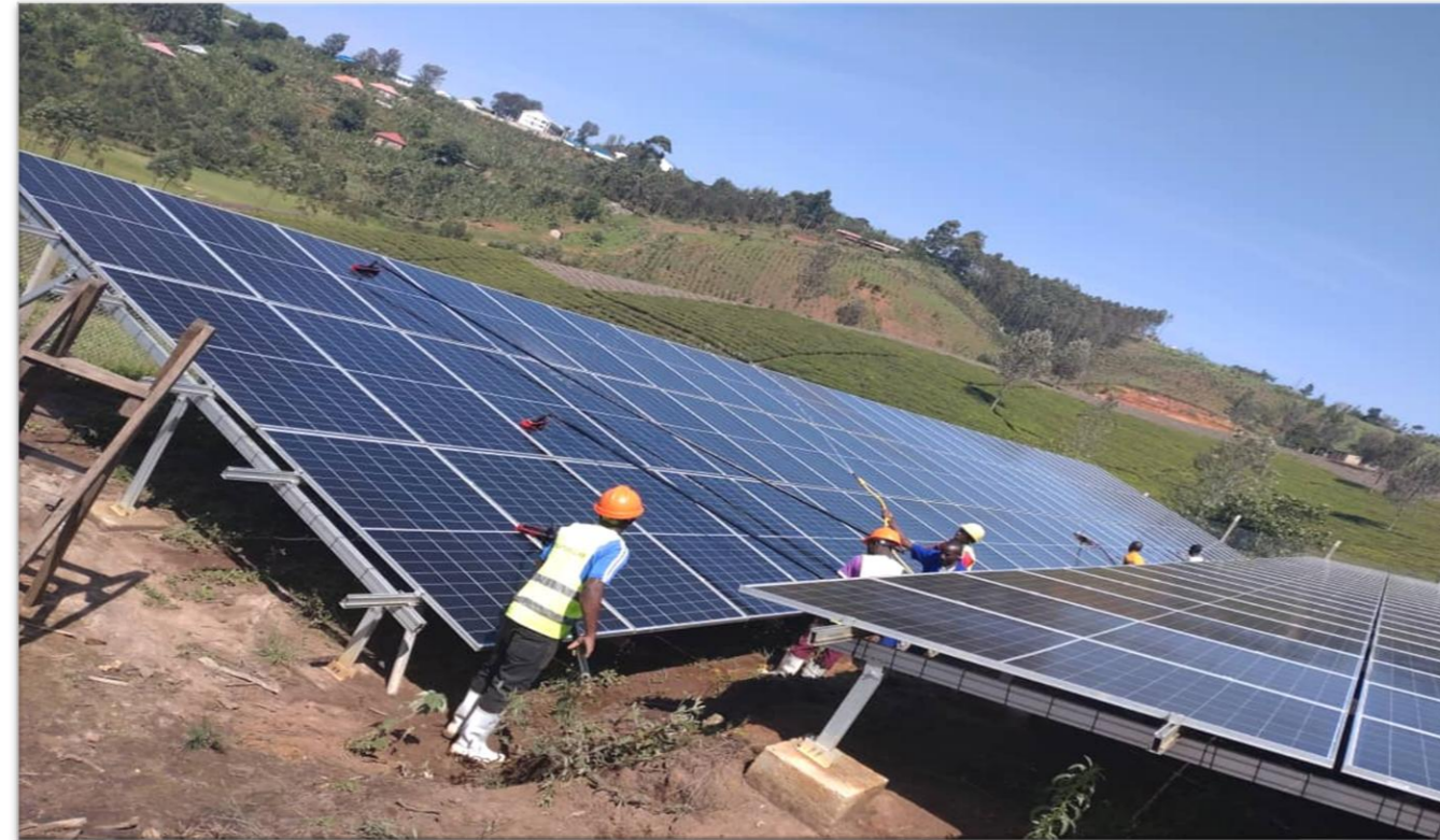
Kyamuhunga Tea Factory: Solar panel cleaning taking place.
