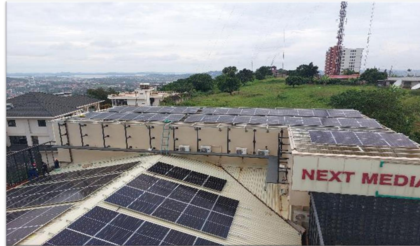
86 kWp Solar PV solution, 96 kWh solar back-up at Next Media Park Kampala.
