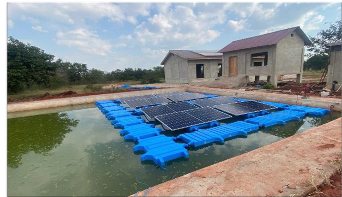
22 kWp and 57 kWh solar system with back up at Sustainable Agriculture Tanzania in Morogoro.
