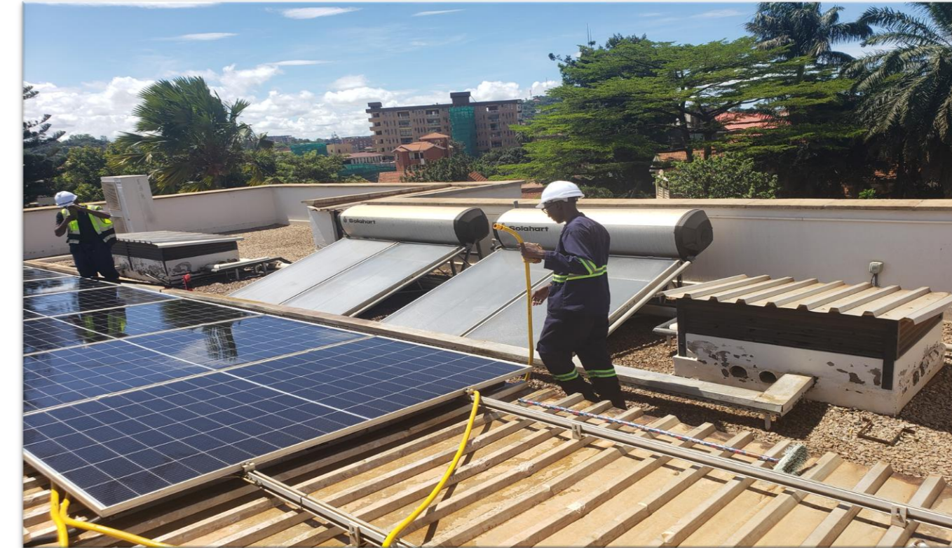
Quality Hill Mall: Solar panel cleaning taking place.
